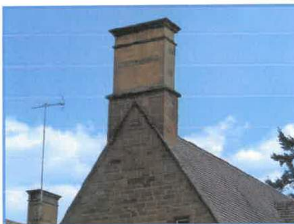
Figure 34 Top: the mixture of historic ridgelines across the village forms part of its character; centre: brick stacks at the apex of the gable end are common in Flore; below: some larger stone farmhouses retain stone chimney plinths, and this example has restored stone stacks.
