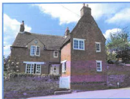
Figure 30 Cob walls can be seen at the grade II listed Adam's Cottage near Chapel Lane. Source: Daventry District Council.
