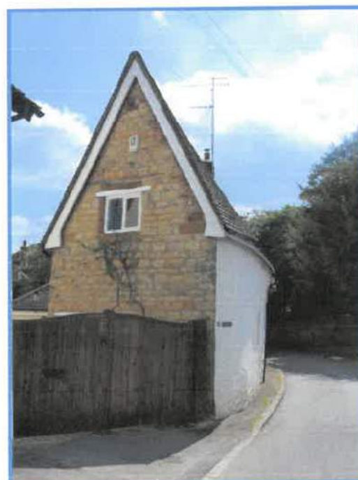
Figure 33 Top: a rare use of render in Flore at Marsh Cottage, with the more common thatch; centre: metal roofing is a local feature where thatch has historically been removed; below: Three Corner House displays a typically steeply pitched roof.
