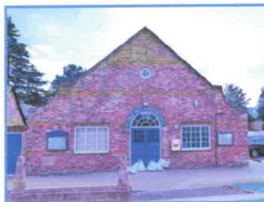
Figure 31 Centre: brick was often used for extensions onto earlier stone properties, as with this polychromatic example; below: Flore Millennium Hall is a local landmark building built in brick in the early 20 th century. Source: Daventry District Council.
