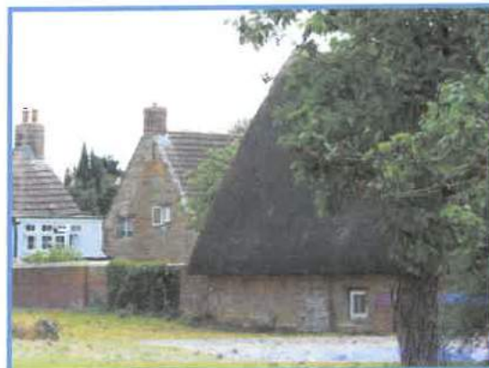
Figure 30 Cob walls can be seen at the grade II listed Adam's Cottage near Chapel Lane. Source: Daventry District Council.
