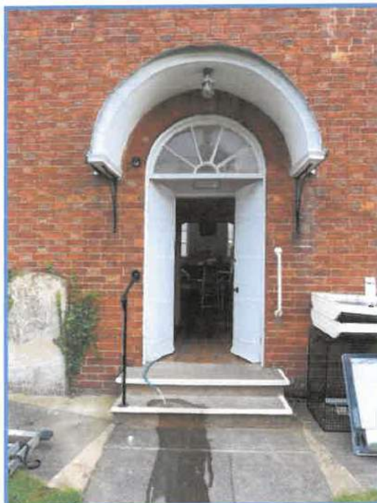
Figure 36 A range of traditional doors across the conservation area.
